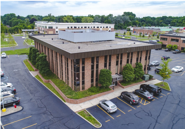
10 West Square Lake Office Building Bloomfield Hills, MI
