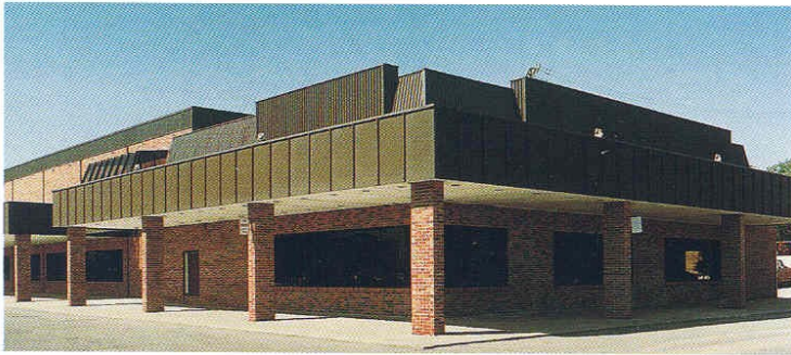
Phase I in Progress
