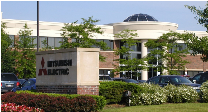
Mitsubishi Electric Automotive in Centennial Business Park Northville, MI
