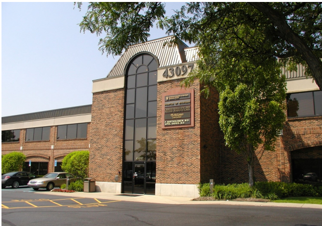
Phase II Completion of Kingswood Office Building
