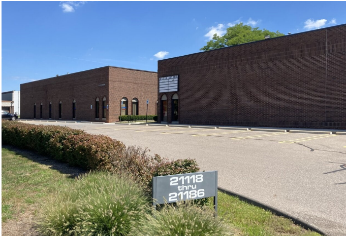
Bridge Commerce Center 1 Southfield, MI
