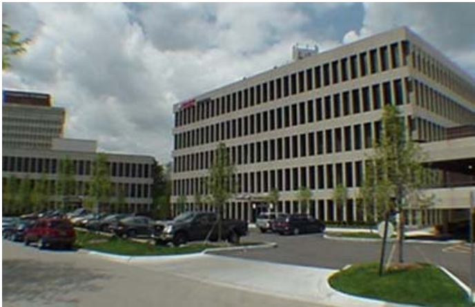
19855 West Outer Drive
